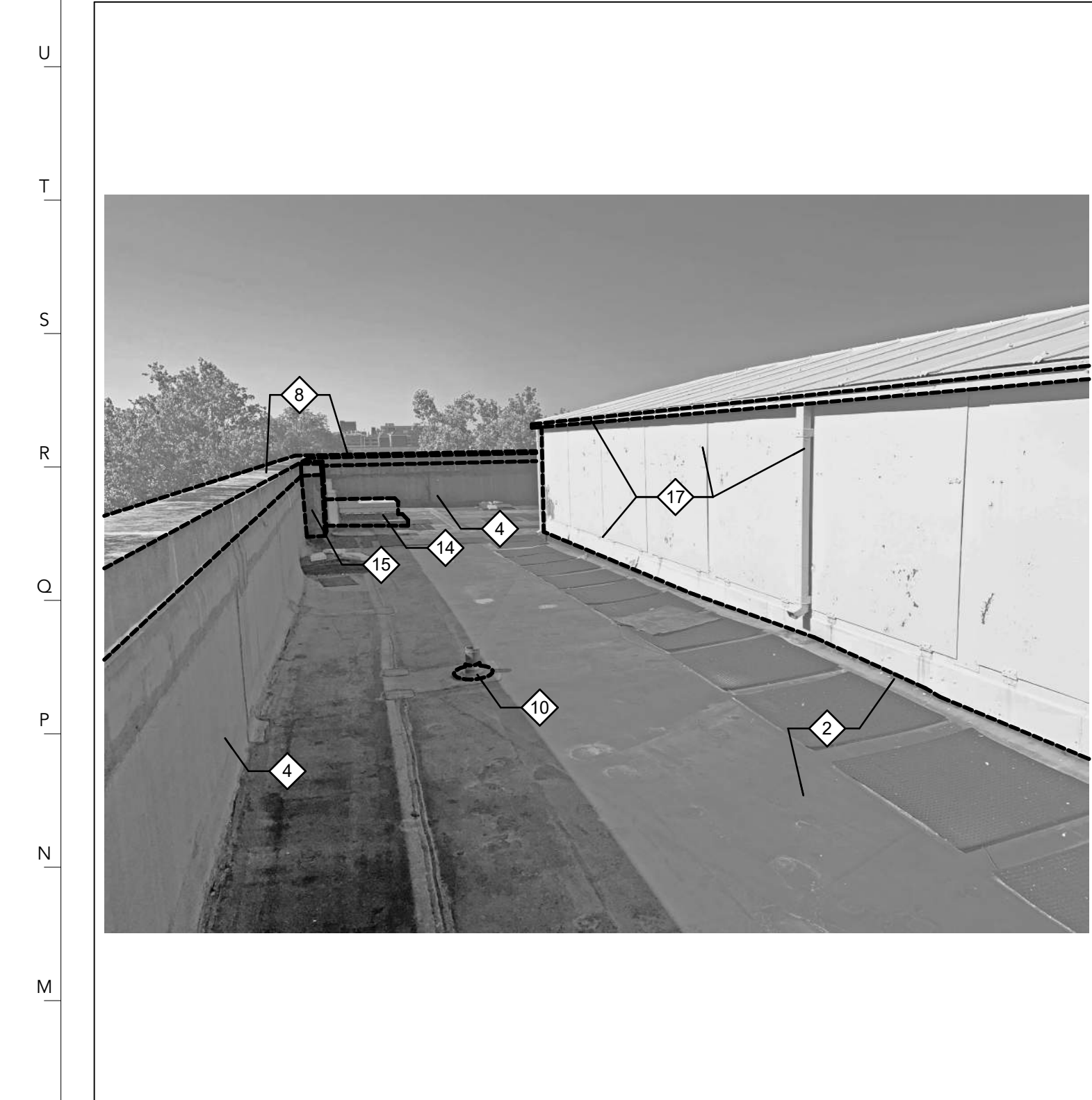
ROOF "B" LOOKING SOUTHEAST | L29
