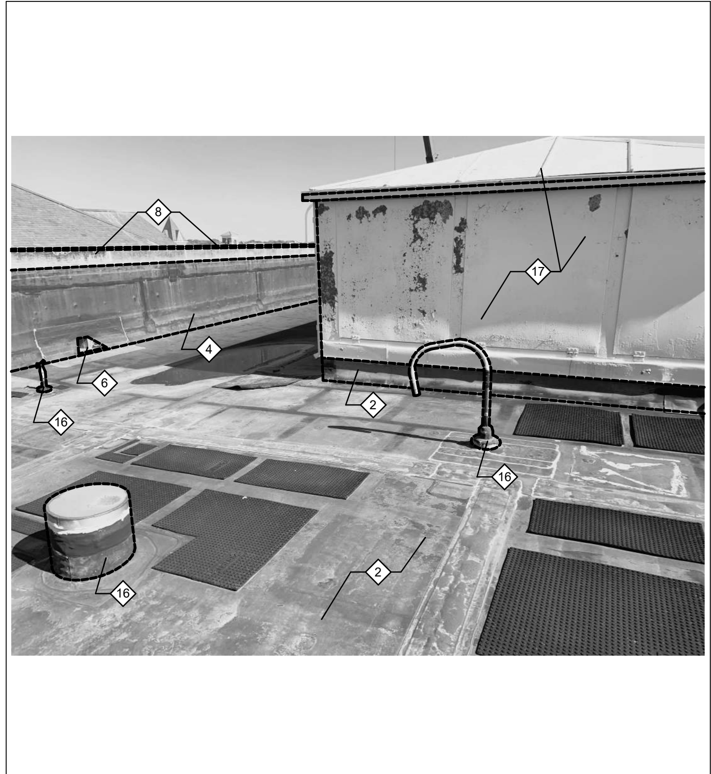
ROOF "B" LOOKING NORTH | L21
